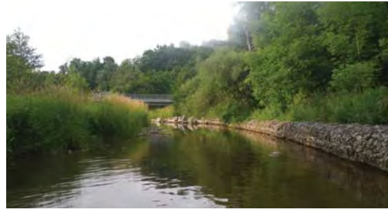
ESMC(1b): Watercourse with undermined gabion baskets
